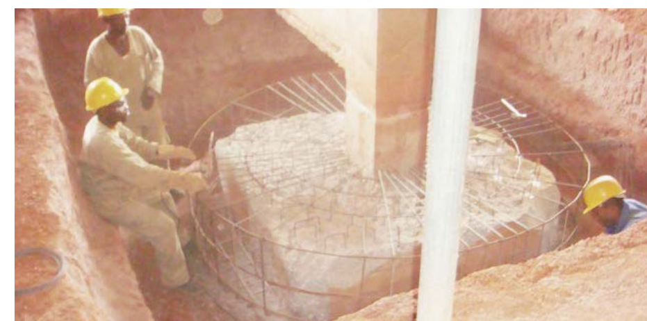
The foundations were strengthened
